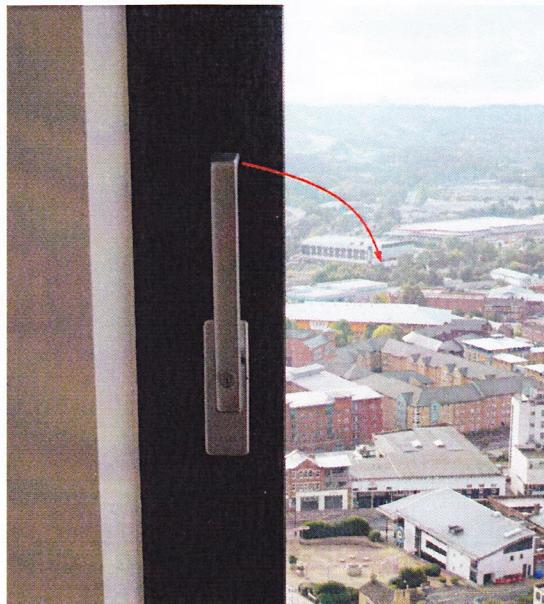
ROTATE THE HANDLE FROM THE VERTICAL POSITION THROUGH 90° AND THE TOP OF THE VENT WILL 'TILT' INWARDS UNTIL IT REACHES ITS NATURAL 'STOP' POSITION
