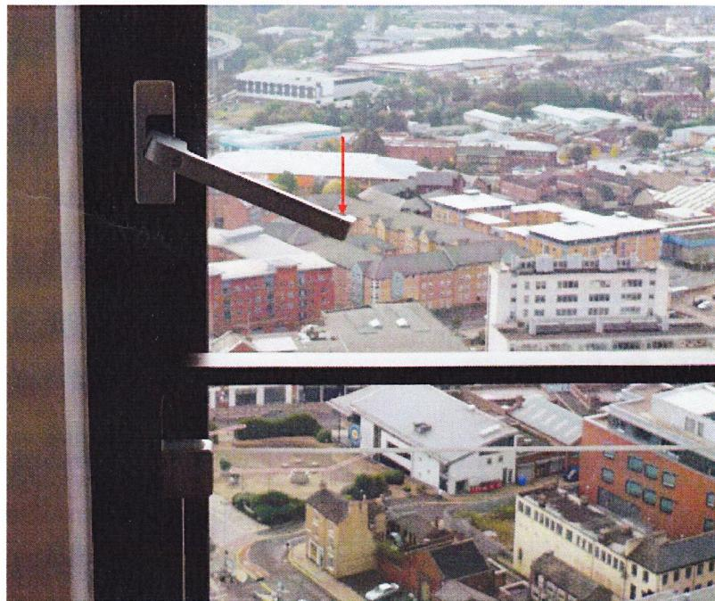
WITH THE VENT IN 'TILT' MODE, MOVE THE HANDLE DOWNWARDS INTO THE POSITION SHOWN ABOVE
